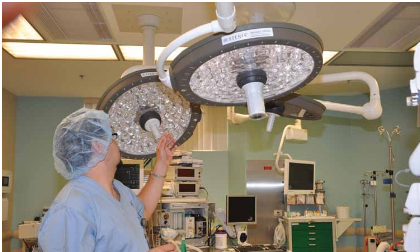
Joe Gallardo, Certified Surgical Technician with VBMC-Brownsville, shows Steris LED operating room lights in the new Surgery suites. The new lights are brighter than conventional operating room lights and generate almost no heat.
